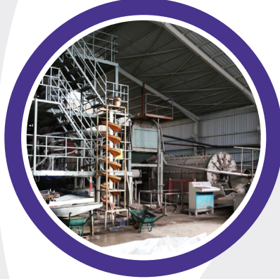
Fabrika Kurulumu Factory Installation
